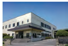
●鹿沼工場：Kanuma Plant
