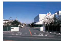
●静岡工場：Shizuoka Plant
