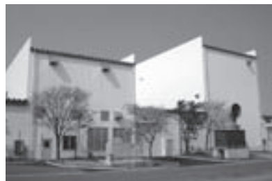
Mass-production facilities at Akita Sumitomo Bakelite Co., Ltd.
