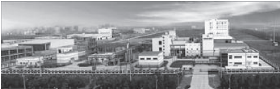
Full view of the plant. The tall building on the upper right is the phenolic molding compound plant.
