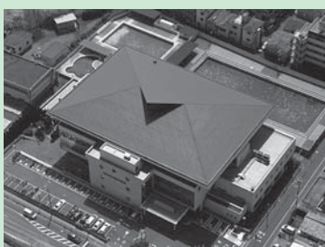
Waterproof sheet used on a building's roof
