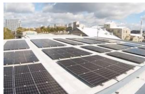
Waterproof sheets with solar anchors
