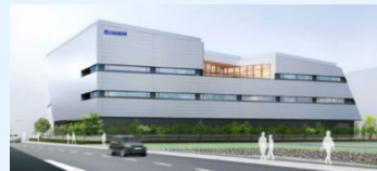
Image of SB-KAWASUMI Head-Office
