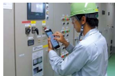
Promoting application of IT to onsite operations (Shift from handwritten inspection reports to entry using electronic terminals)
