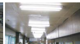
All fluorescent bulbs in offices have been replaced with cold-cathode fluorescent lamps.
