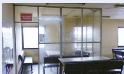
Partition separating smoking/non-smoking sections (PT. SBP Indonesia)
