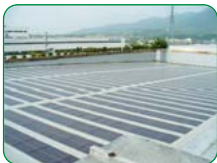
Installation of photovoltaic facility (Nara Plant)
