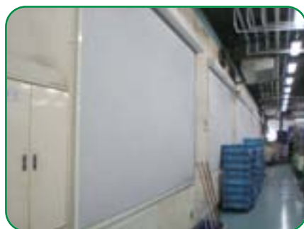
Light shield installation (Tsu Plant)
