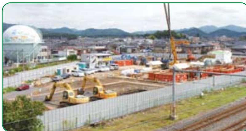
Overall view of purification facility construction site
