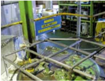
Safety fence installed above mixing tank (Shizuoka Plant)
