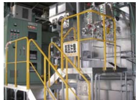
Boiler converted to utility gas (Amagasaki Plant)
