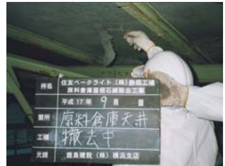
Asbestos removal
