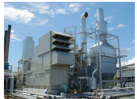
Cogeneration system (Shizuoka Plant)
