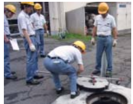
Drill on blocking wastewater leakage (Fundamental Research Laboratory)
