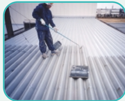
Heat-insulating paint on plant roof
